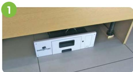
Remove the kick board from the kitchen and the front cover from the Sweepovac. Slide the Sweepovac unit into location.
