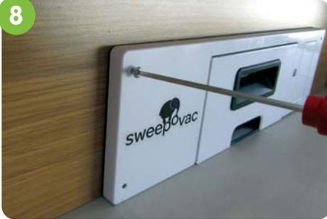
Attach the front face plate using four M4 x 10mm hex screws (included).
