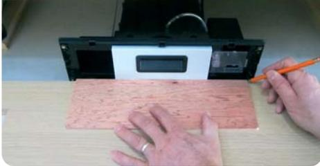
Remove the front panel from the Sweepovac unit. Place the template on the kickboard in the centered location as shown. Draw a line around the 3 sides.
