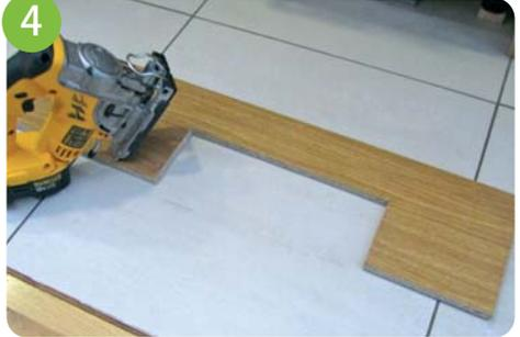
Use the jigsaw to accurately cut along the center of the line
